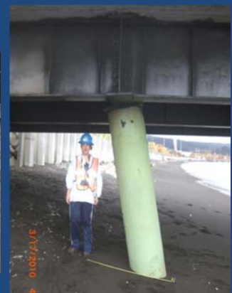
Coronel : Settlements / Displacements, Sand boils, Piles damage
