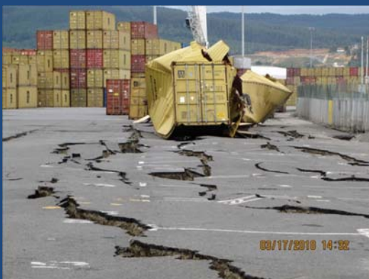
Coronel : Settlements / Displacements, Sand boils, Piles damage
